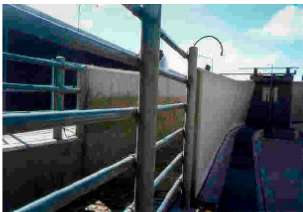
Fig. 12: Curved cattle race with solid sides
