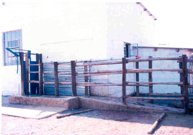
Fig. 45: Simple, effective race and neck crush for cattle restraint
